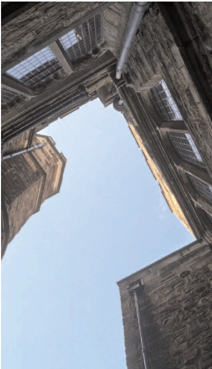
Looking up from behind the Servery
